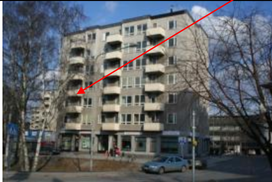
Figure 1a. Kommunalvägen 20, Entrance towards west.
