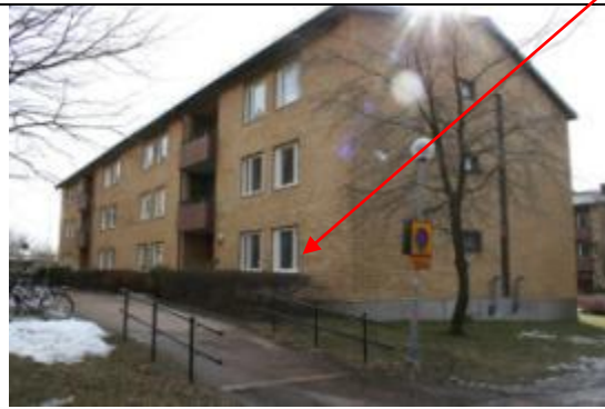
Figure 1a. Rosenborgsgatan 24 A, entrance.
