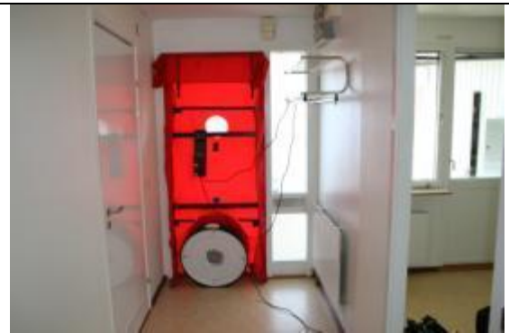
Figure 2. Blower Door placed in opening for front door, gives the under pressure -50 Pa during testing.
