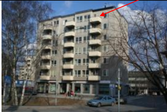
Figure 1a. Kommunalvägen 20, Entrance towards west.
