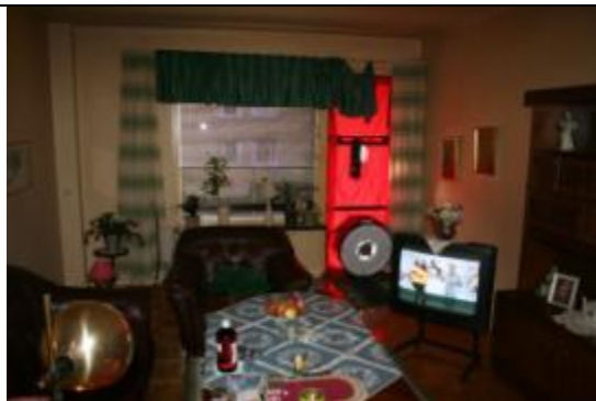
Figure 2a. The Blower Door was mounted at the balcony door opening.
