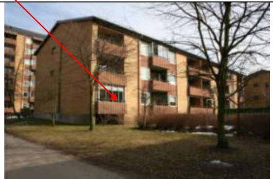
Figure 1b. Rosenborgsgatan 24 A, balcony side.
