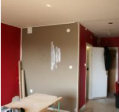
Figure 8a. The apartment has, exhaust air devices both in bath room and living room.
