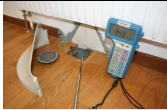
Figure 10b. In the second floor opening in the living room was an air speed of 3,4 m/s measured, corresponding to about 15 l/s.
