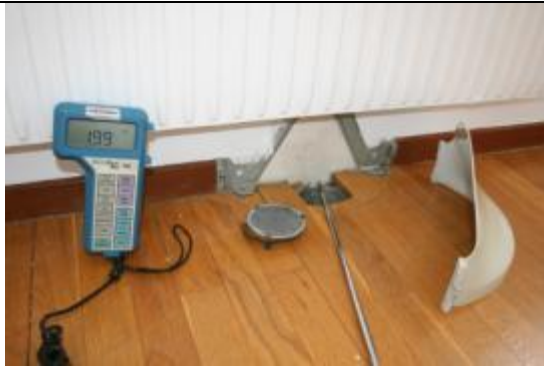
Figure 10a. In living room were 2 m/s measured in the opening, corresponding to about 9 l/s.
