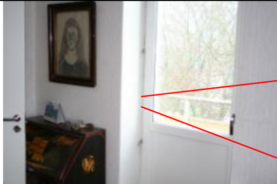
Figure 6a. Balcony door.
