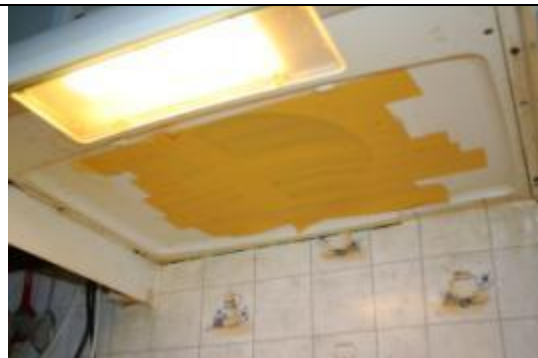
Figure 2a. At air tightness tests was the hood temporarily tightened.
