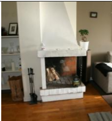
Figure 5a. Air tightness testing were performed both with sealed stove and unsealed stove. The smoke damper was closed in both measurements.
