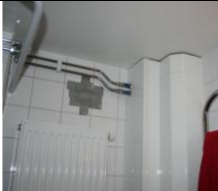
Figure 10a. The biggest leak was found at mounting for water pipes. Probably is fire tightening between pipe and structure untight and air may be overflow between apartments. The tenant has problem with smell of smoke from the neighbor.
