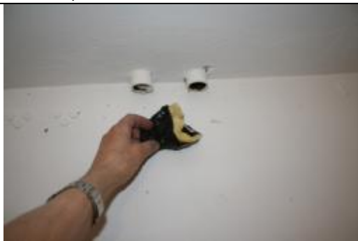
Figure 7a. The pipes were temporarily sealed with glass wool.
