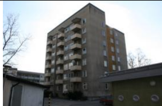
Figure 1b. Kommunalvägen 20. Facades towards east and north.
