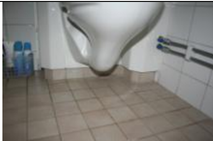
Figure 10a. The biggest leak was found at mounting for water pipes. Probably is fire tightening between pipe and structure untight and air may be overflow between apartments. The tenant has problem with smell of smoke from the neighbor.
