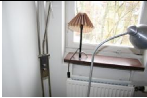
Figure 5a. Leak between windowframe and arch.
