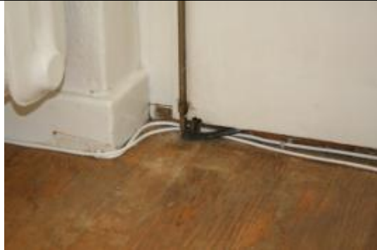
Figure 2a. Leak at balcony door, between arch and door frame/step.
