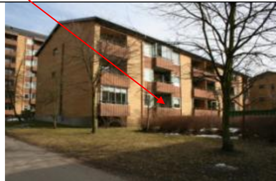
Figure 1b. Rosenbergsgatan 24 A, balcony side.
