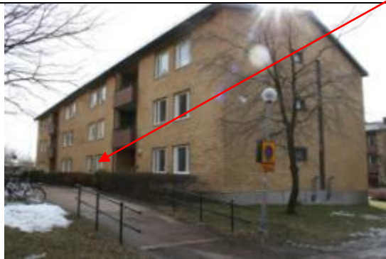
Figure 1a. Rosenbergsgatan 24 A, entrance.
