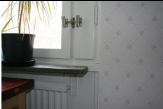
Figure 6a. Kitchen, airing window.
